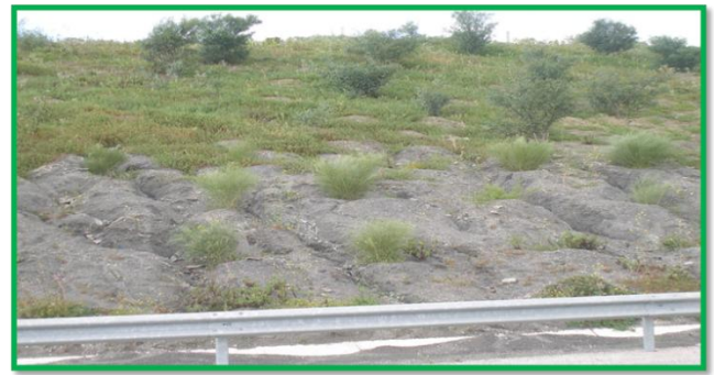
Figure 9. Spatial Dynamics of Gully Erosion Along the Tangier–Tanger Med Port Motorway Corridor
