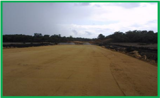
Figures 6 and 7. Forest clearing in Dar El Foual Forest during the construction of the Tangier–Tanger Med Port Motorway
